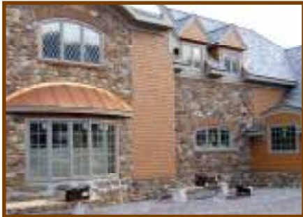
Copper Standing Seam Bay Window
