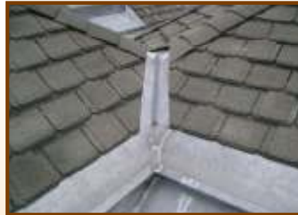
Lead-Coated Copper Valley & Pool Gutter
